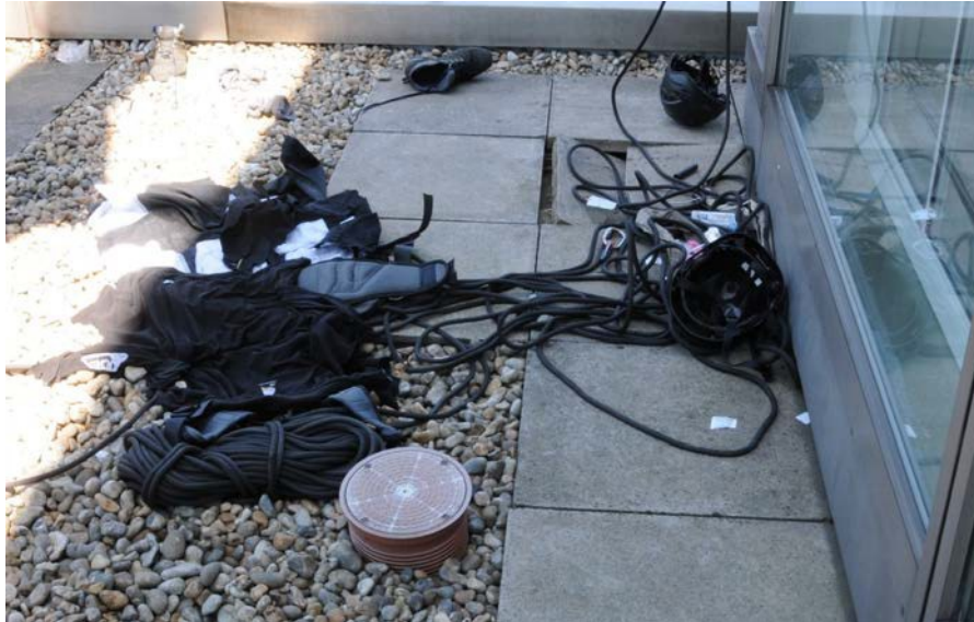
Photo 1: Broken slab where injured person landed during fall
