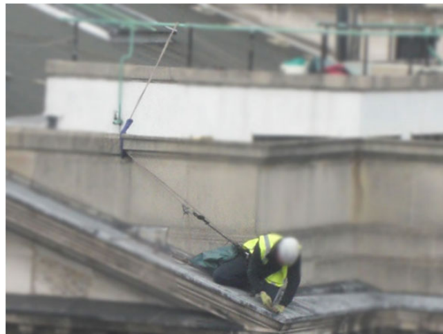
Figure 2 - Poor anchor selection and anchor lines positioning. Reliance on an unproven handrail. Risk of a swing fall.
